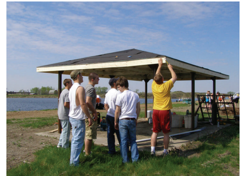
Students renovating picnic shelter.
