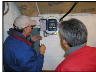
Installation of data logger at Epping, ND tower site.
