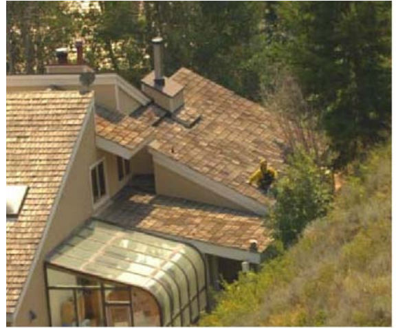
Local firefighters completed REDZONE assessments at high risk rural homes.
