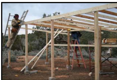
Hank Stevens constructing a raincatcher.
